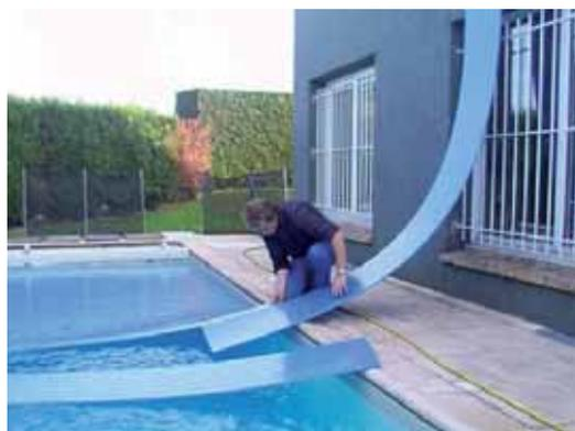
USING A MALLET, CLIP THE LAST FEW CENTIMETRES TOGETHER WHILE HOLDING THE SLATS AT A 45° ANGLE
